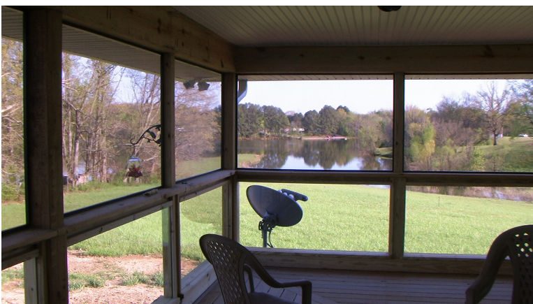
Contractor Steve Donnelly installed the MINI Track™ Porch Screening System on his sister's 1,920 square foot home on Old Hickory Lake in Hartsville, TN.
